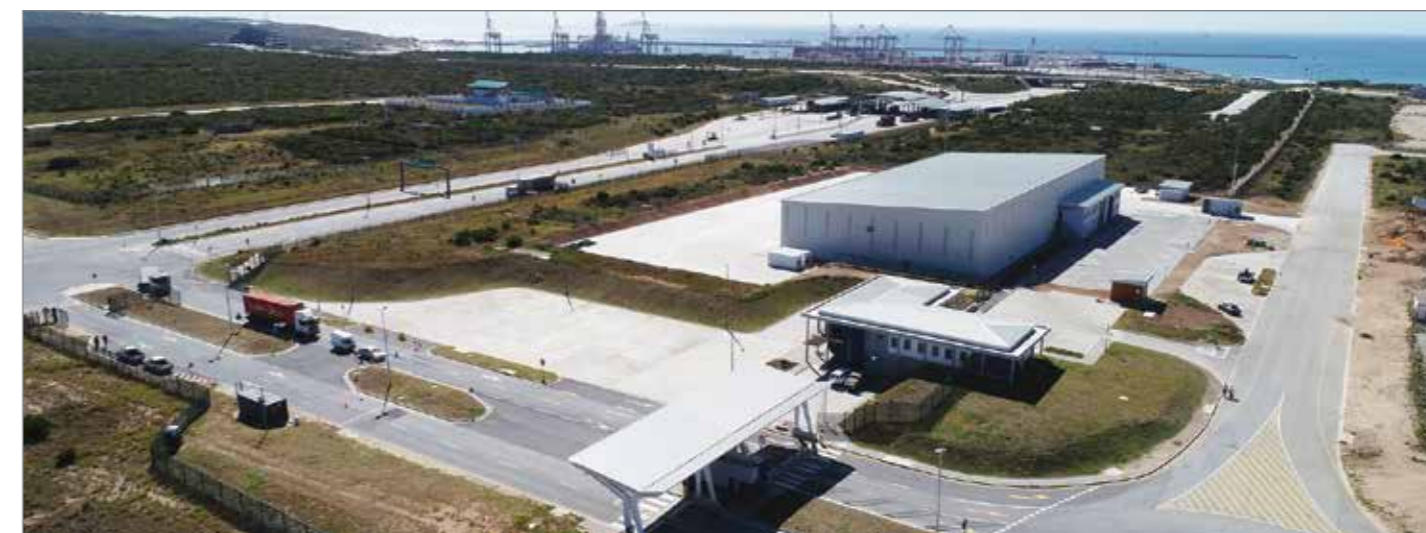
CUSTOMS CONTROL AREA – WAREHOUSE IN ZONE 1.
