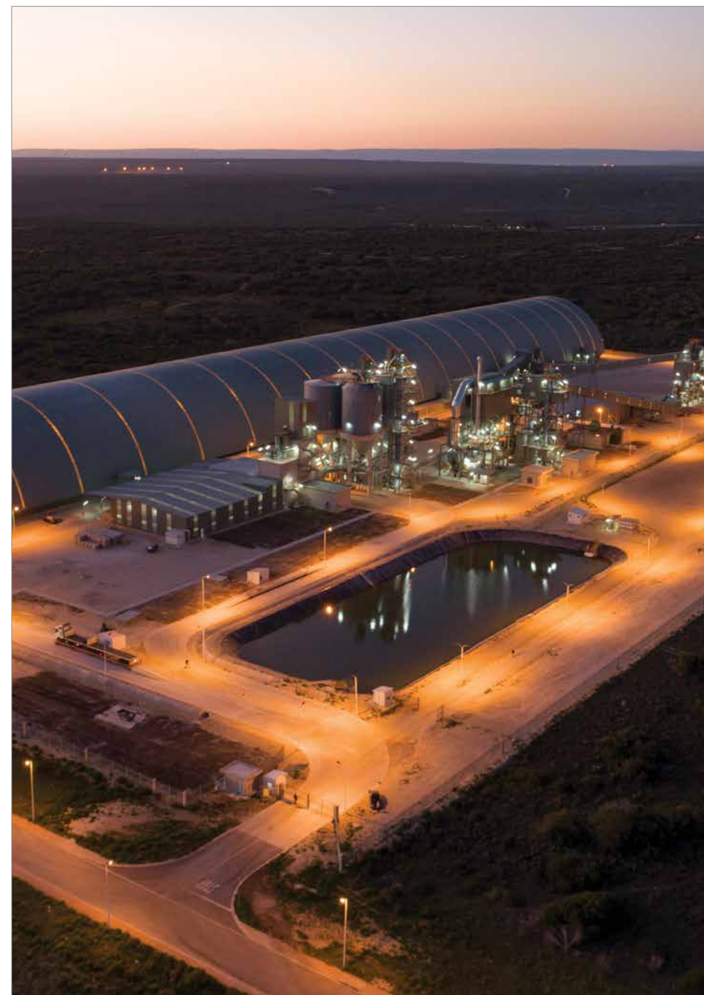
CEMZA CEMENT FACTORY AT DUSK.
