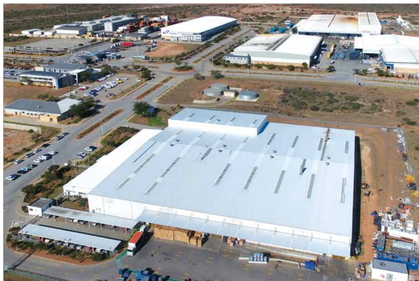
The purpose-built Nelson Mandela Bay Logistics Park (NMBLP) in Uitenhage is managed by the CDC.
